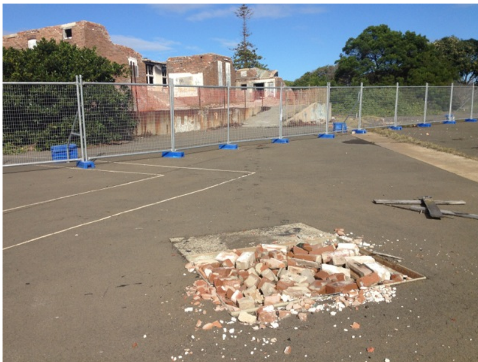
Photograph 2 – Previous main building, located in the centre of the site, and suspected septic tank area. Photograph taken in August 2013 before the building was completely demolished.
