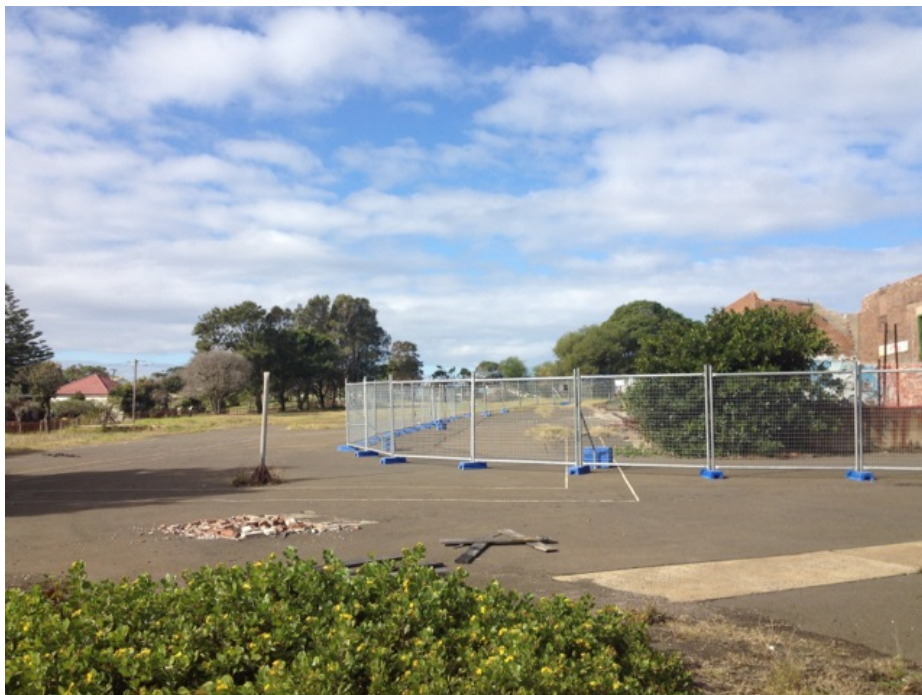
Photograph 1 – Previous main building, located in the centre of the site. Photograph taken in August 2013 before the building was completely demolished.
