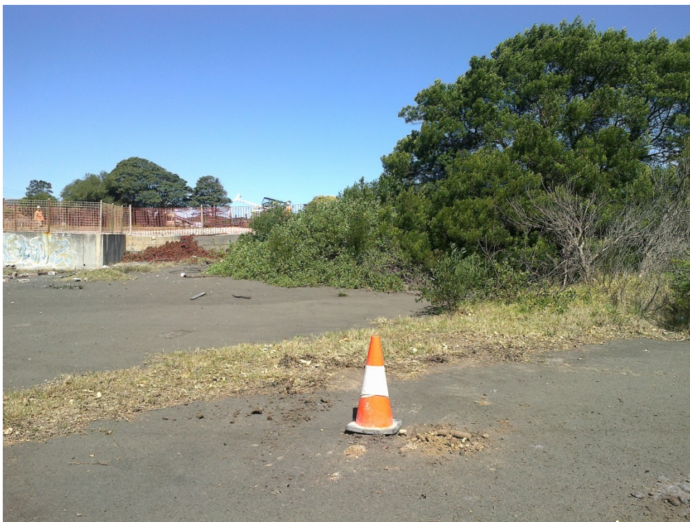
Photograph 5 – Photograph shows location of BH4/ MW4. Photograph taken during the second stage of works, October 2013, after the main building was demolished.
