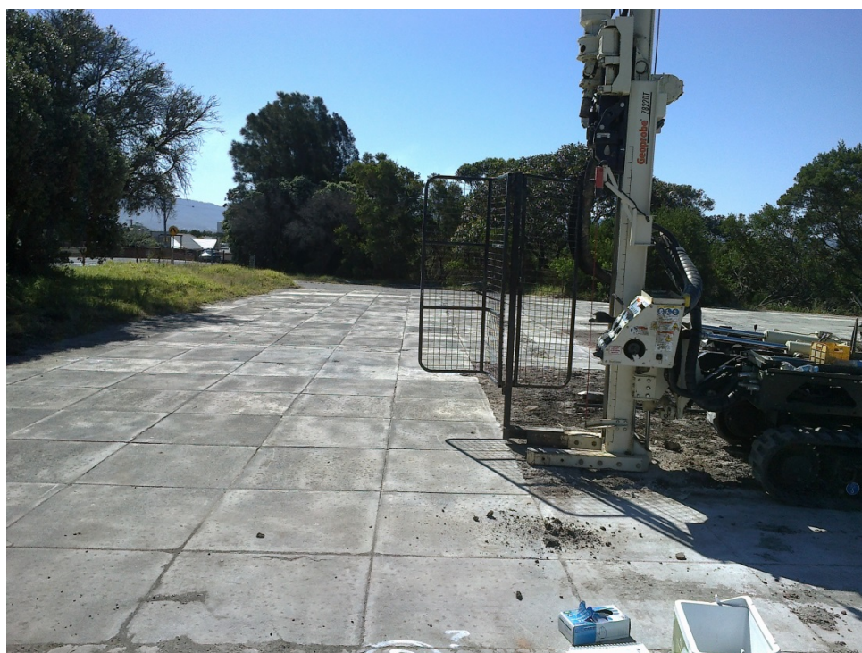
Photograph 6 – Borehole BH2 at the location of the former main site building, in the centre of the site. Photograph taken during the second stage of works, October 2013
